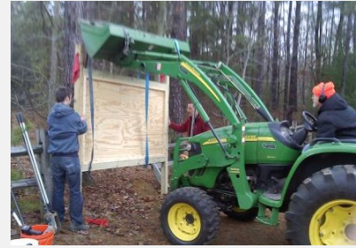
Sean Cartwright, Pieter Litchfield and David Rathbun installing new kiosk.
