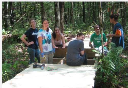
Skidmore Student Conservation Corps members building boardwalk.
